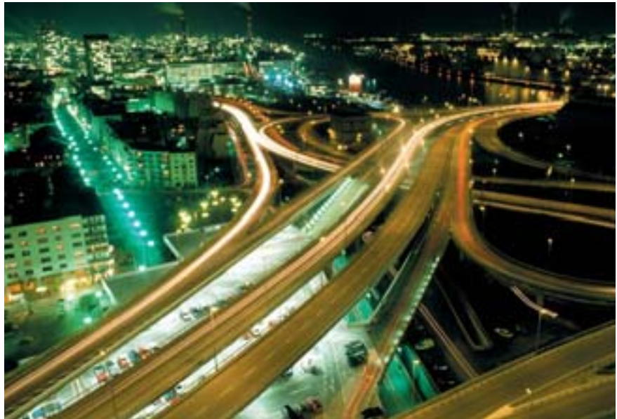
Motorway system in Ludwigshafen, Germany© Maximilian Stock LTD/SPL/Cosmos
